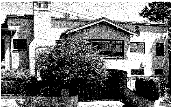
The west side of the house still has the original vertical folding garage doors, in good condition. You can also enter the basement through a back door. To the right is the house the Martins lived in before they built this one.
